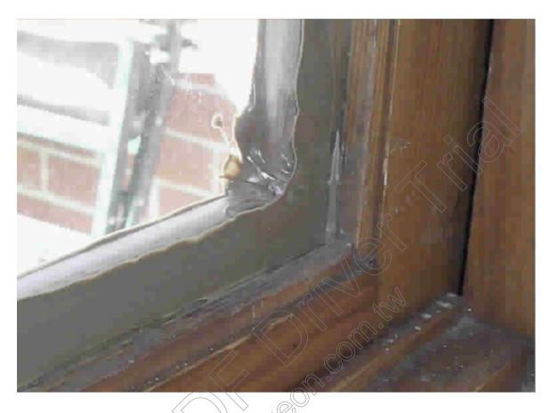
No, it's not Lindor chocolate, this is excess brown butyl mastic making sure of a good seal at the butt joint. Despite the brown colour scheme, appearances would be improved by the use of wooden beading or mouldings to hide the glue, and ensure that the glass cannot become unstuck.
