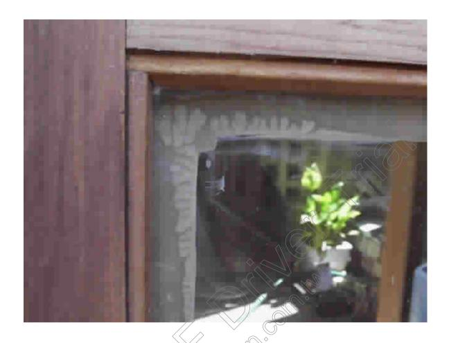
If the plastic extrusion in not perfectly straight, then it can slowly lever the sheets of glass apart, and break the airtight seal. Surprisingly this window has had a failed seal for over tewlve months, and still no condensation has appeared in the air-space.
